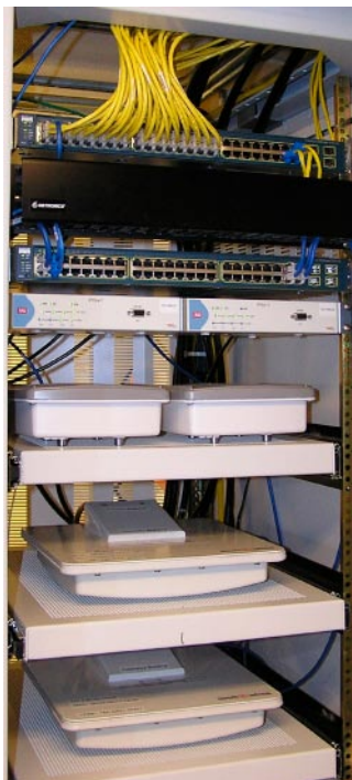
CSBF communications rack – PTP 400 Series radios, IP-MUX, WLAN, etc.
